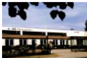
AKG Thermotechnik GmbH & Co. KG Uslar, Germany
